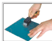
step 1: make grid cutting on surface
